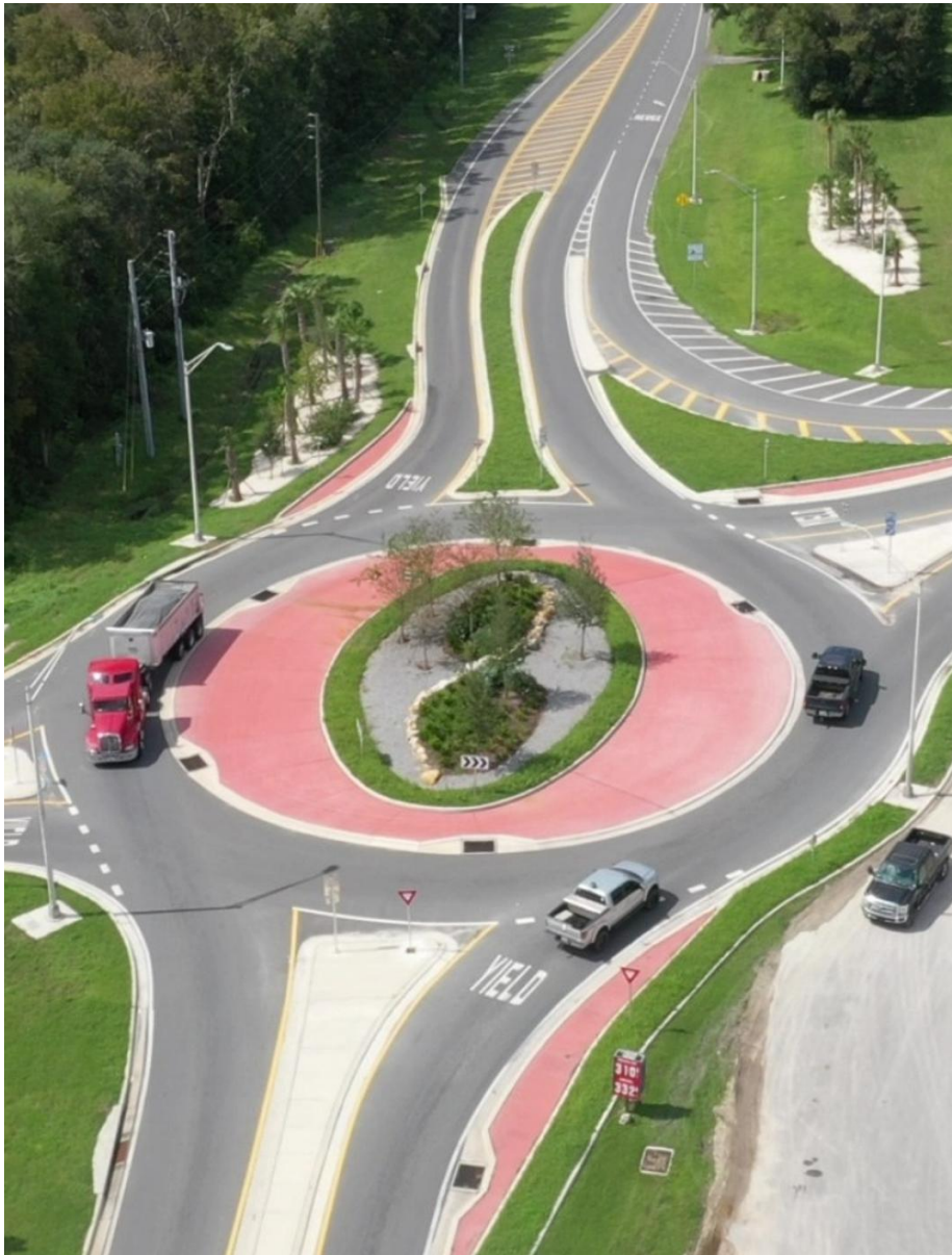
A single-lane roundabout completed in 2023 in Hernando County improves freight operations and safety conditions for all roadway users by reducing turning constraints for large vehicles and eliminating sight distance concerns. (Photo Credit: Benesch 2024)
