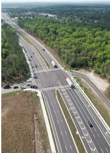
Figure 4 – Improvements to Add Capacity and Correct Truck Turning Issues at US 98 / SR 50 / Cortez Boulevard and Kettering Road in Hernando County
