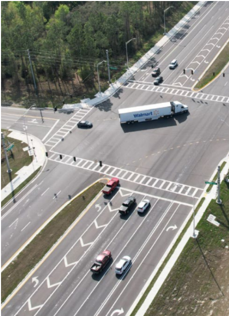
Figure 4 – Improvements to Add Capacity and Correct Truck Turning Issues at US 98 / SR 50 / Cortez Boulevard and Kettering Road in Hernando County
