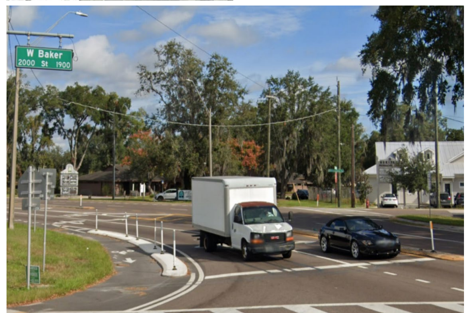
Figure 5 – Intersection Improvements to Facilitate Trucks Turning Movements at US 92 / SR 600 and SR 566 / Thonotosassa Road in Plant City
