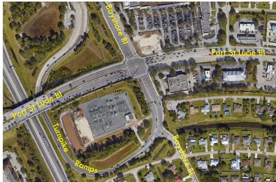
Figure 5.3 Port St Lucie Blvd at Bayshore Blvd
